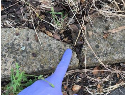
Figure 11: metal item in ground at front
